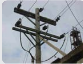
Distribution line faults
