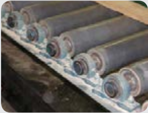
Overheating conveyor bearing
